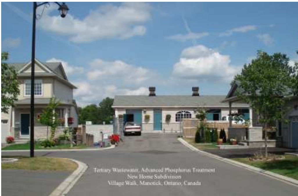
Ottawa Ontario: Manotick Wastewater Treatment Plant
