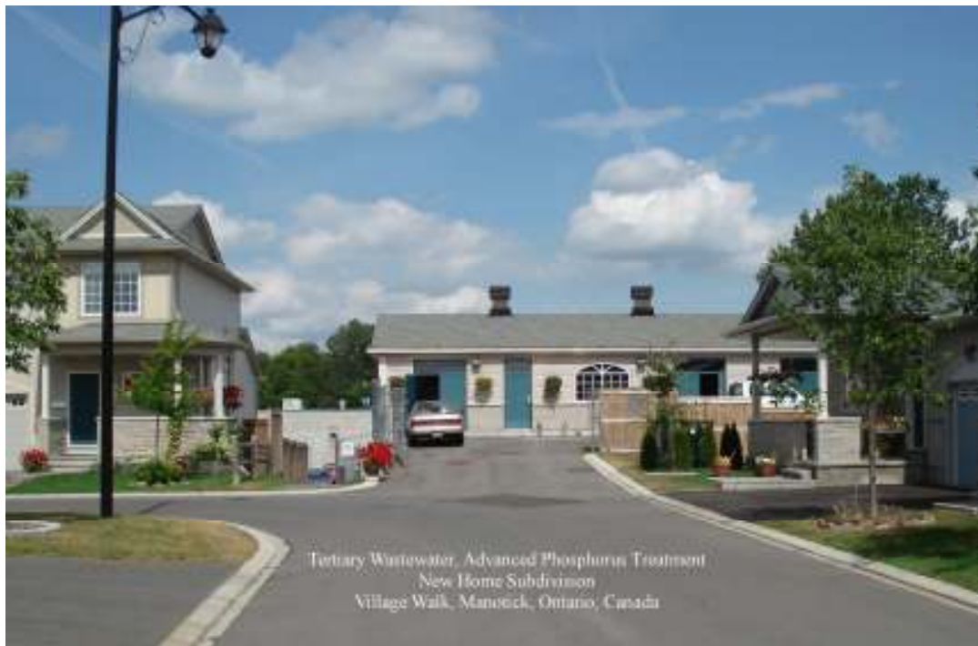
Manotick Ontario Advanced Tertiary Wastewater Treatment Plant
