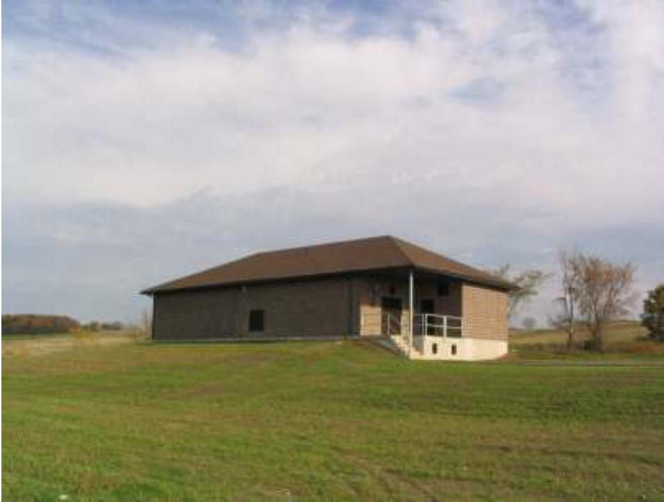
Tertiary Wastewater Plant: 200 Home Subdivision North of Toronto
