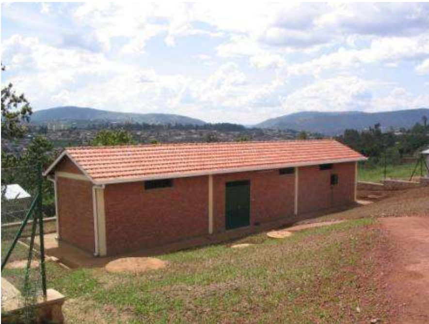
Rwanda Africa: Tertiary Wastewater Plant for 450 Homes
