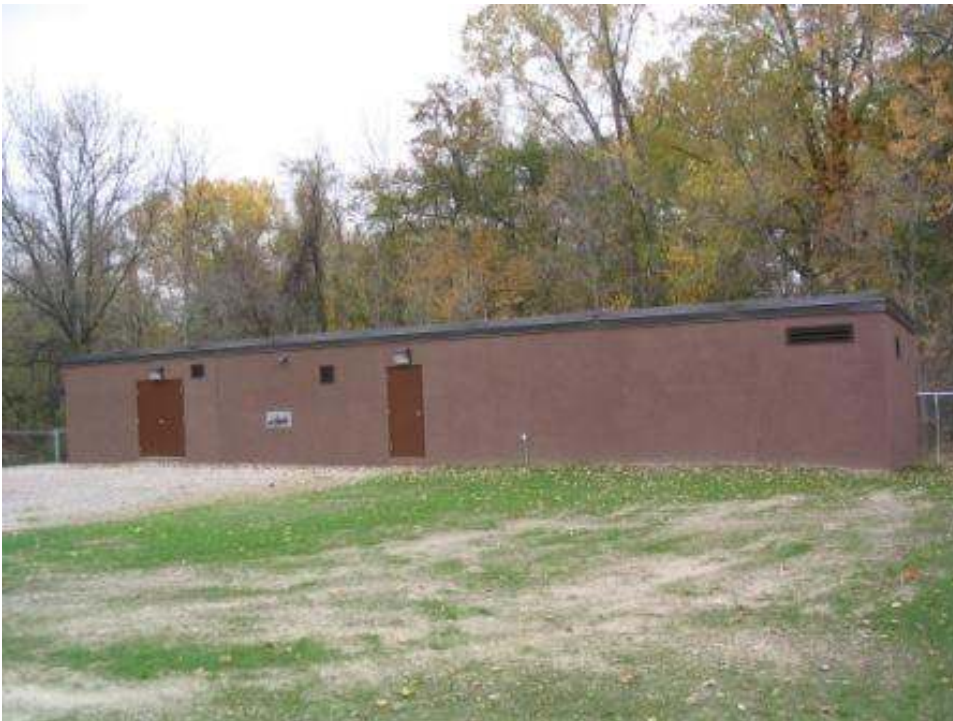
Town of South Woodlee: Tertiary Wastewater Treatment Plant
